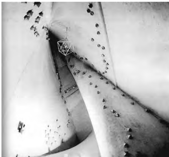
Figure 2: Sound paths created by hundreds of pyramidal speakers placed in the interior of the Philips Pavilion
